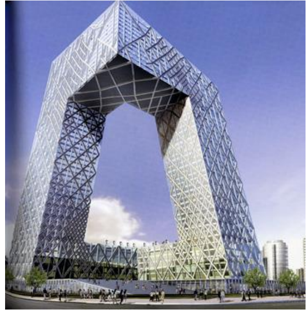
Figure 1.2 – China Central Television Building, China
