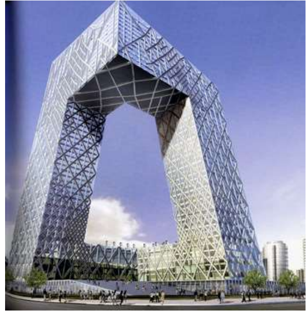
Figure 1.2 – China Central Television Building, China
