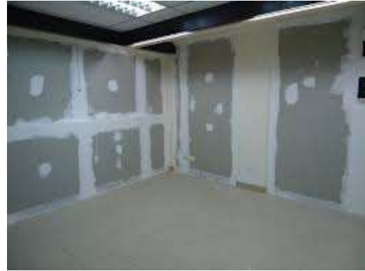
Plaster Boarded Walls
