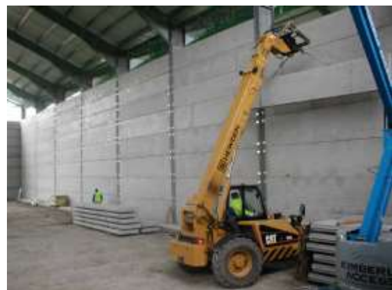
Fitted Wall Panels
