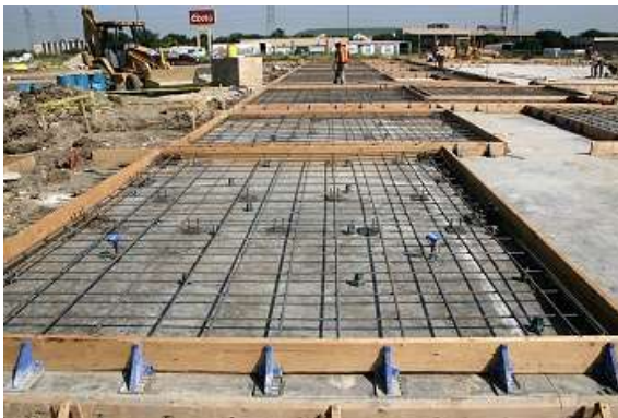
Tilt-Slabs on Floor Ready for Pouring
