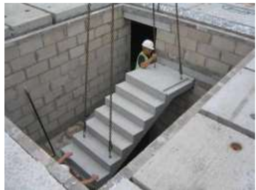
Stairs being Installed
